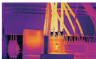
Electric Routine Inspection
