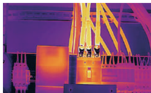
Electric Routine Inspection
